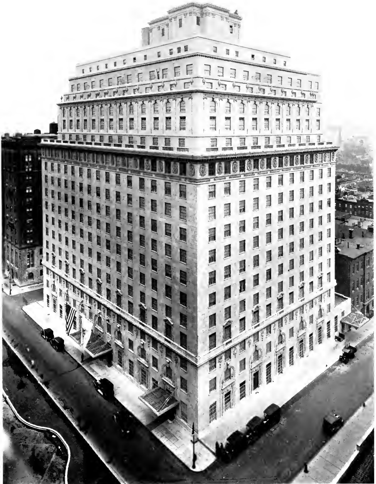
THE AMBASSADOR HOTEL, PARK AVENUE, NEW YORK VIEW FROM SOUTHWEST WARREN & WETMORE, ARCHITECTS
